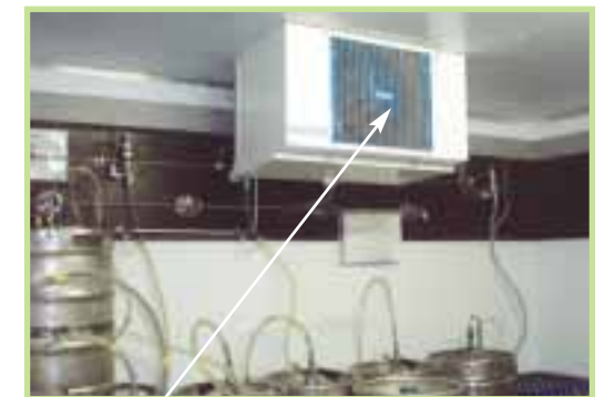
Keep evaporator fins clean
